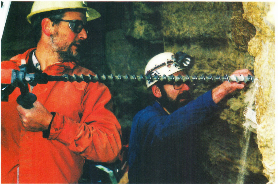
G Heavy drilling work for installation of the access ladder.
