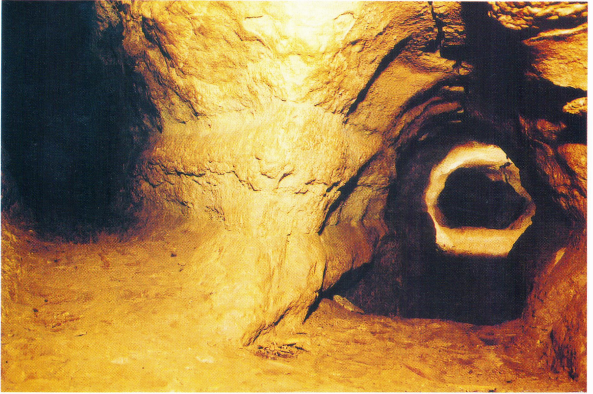
F Usual gallery profile, with silt layer covering the floor.
