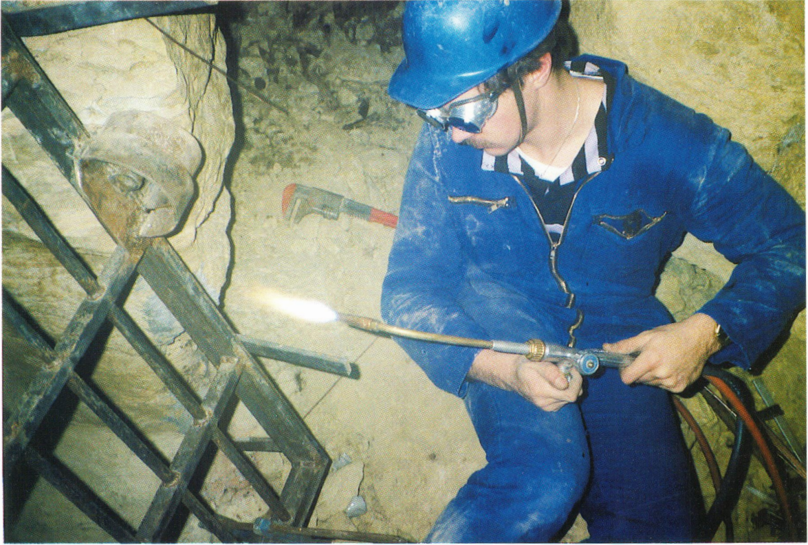
H Welding the entrance door
